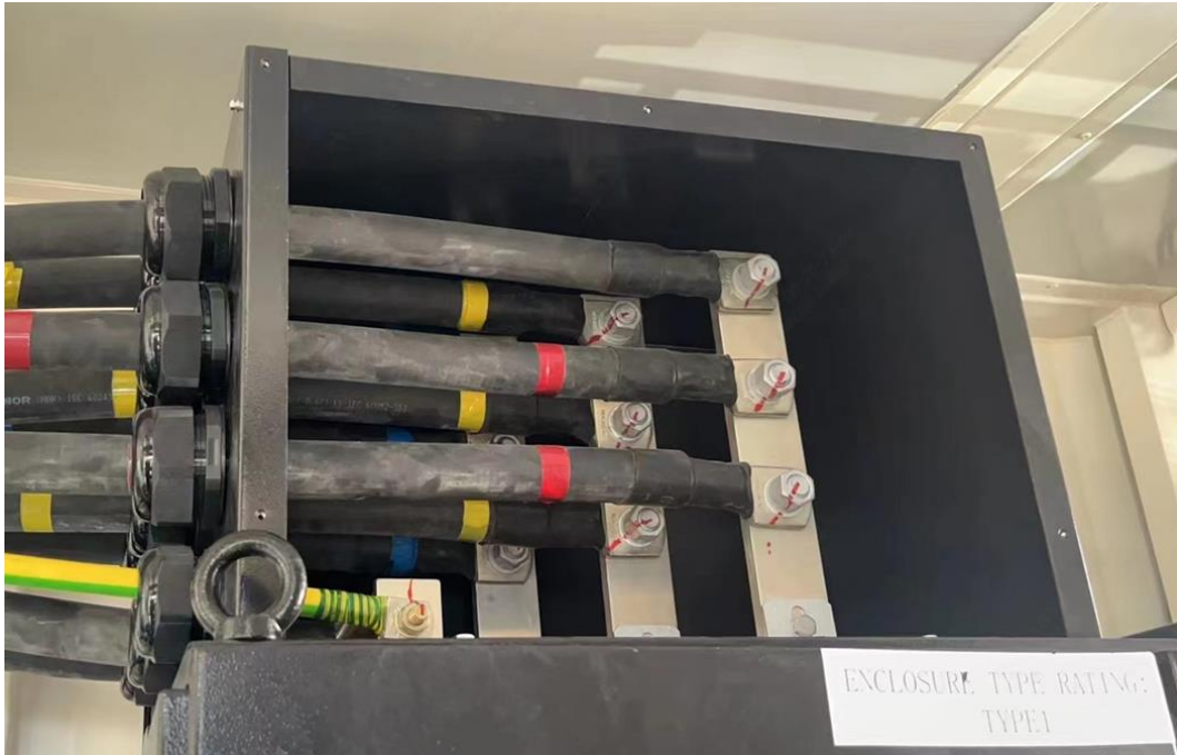
Figure 7-20 Cable connection diagram
